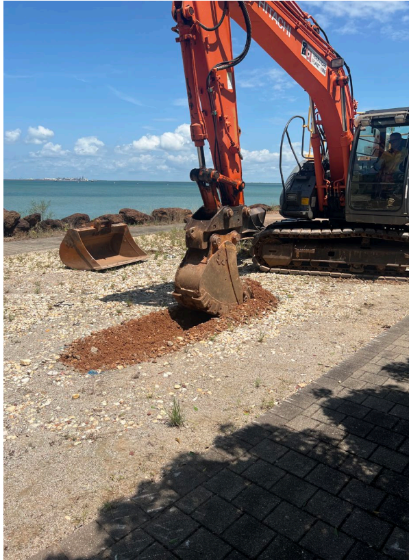
Images from SLR's work on the LCC site: making the sample bores and an example of some of the sample bores.
